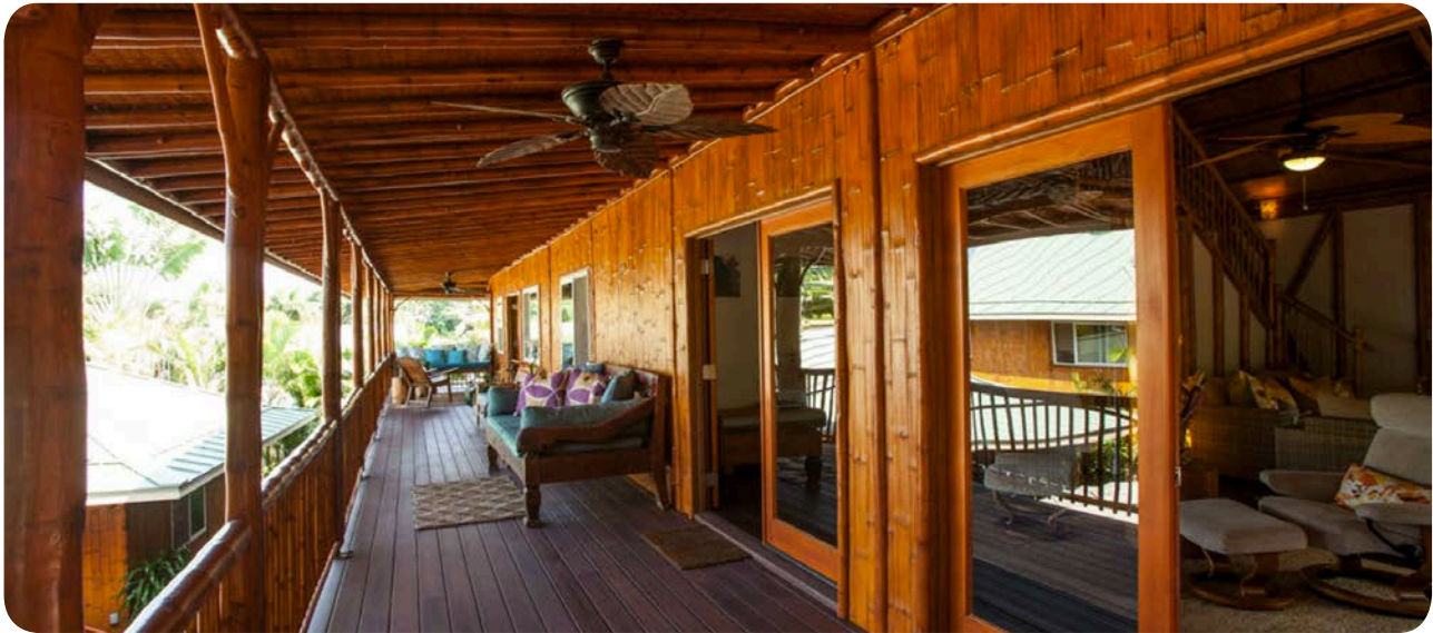
Signature Polynesian 1619 front porch with split bamboo exterior siding, bamboo porch posts, railing, and pickets.
